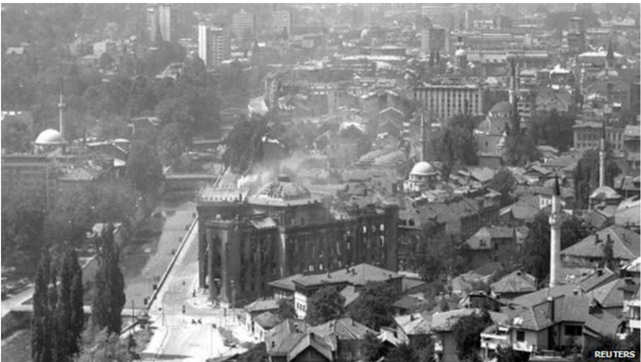
Fig. 4. Sarajevo's National Library. The iconic building was hit by a mortar and burned down during the Bosnian Serb siege of the city. Almost two million books were destroyed after the building's shelling and fire in August 1992.
